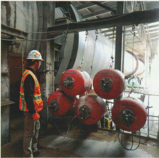
Workers are able to access the tanks in a safe and comfortable area, with ample room to work.
