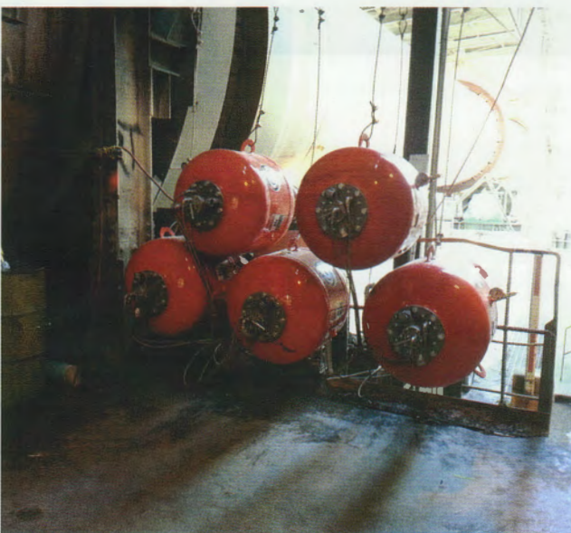
Valves face outward for convenient maintenance, requiring no tank removal to service them.
